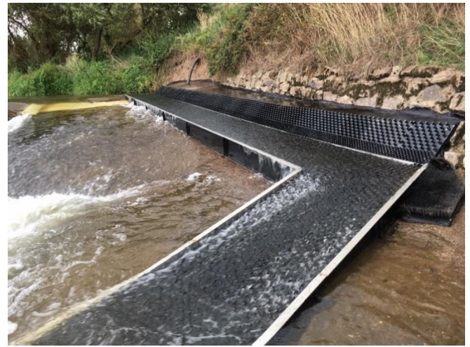
Left, thousands of eels attempt to migrate up Tewkesbury weir, River Severn, UK. Right, an eel pass constructed in 2018 allows them to migrate.
