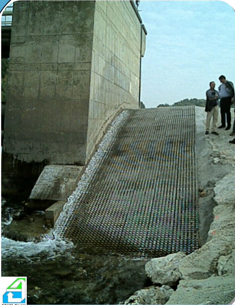
Eel ladder with concrete plot substrate
