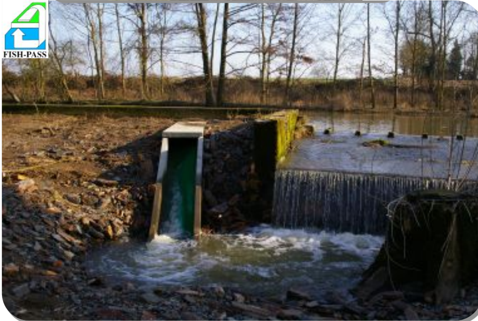
Prefabricated gutter with brushes substratum
