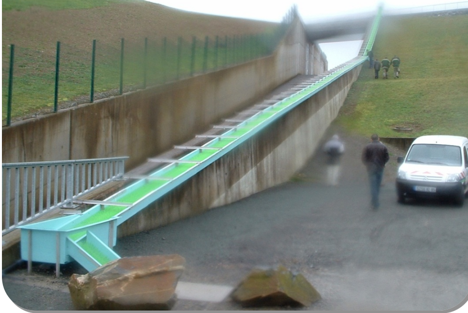
Modular eel ladder with counting facilities for high dam
