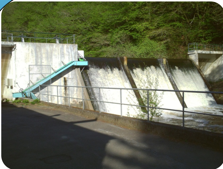
Dam equipped with a prefabricated gutter
