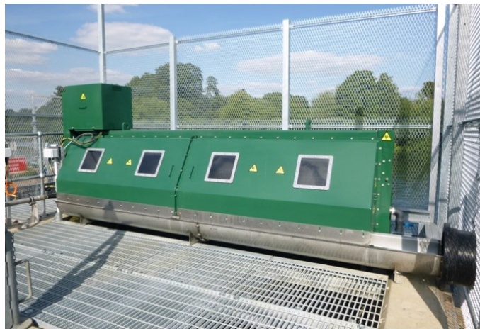
Hydrolox traveling water screens operating at Affinity Water Limited's Chertsey water treatment location.
